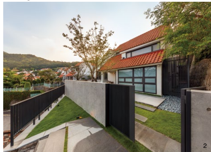
2. 外觀，利用圍牆與斜坡，維繫住宅隱私。3. 餐廚空間，斜面天花板與開放感，空間線條簡潔卻深具張力。4. 餐廚空間，視野能放望至庭園、客廳以及泳池區，時時關照家人動態。5. 餐廚空間，設在採光最佳處，水泥粉光與清水模獨有的質感與紋理，在光色之中更顯飽滿，既純粹又豐富。 2. Exterior view is a topographical feature. 3. Dining/kitchen. 4. Dining/kitchen and great view toward garden, living room and swimming pool. 5. Dining/kitchen enjoys great natural light and surrounded by good texture furnishing.
