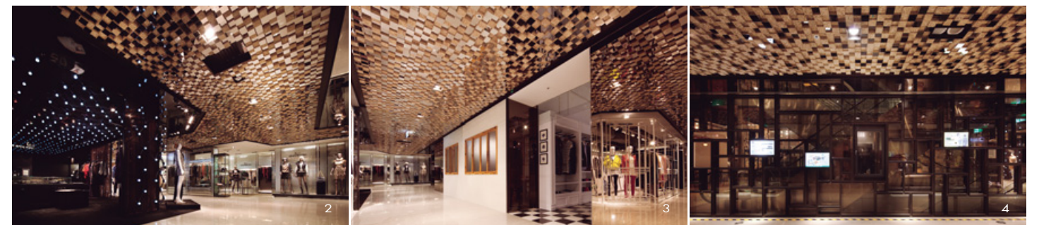
1-4. B1，運用鑽泥板與不鏽鋼拼出立體格紋，不鏽鋼鋪面由疏至密的漸層編排，產生像素化的視覺效果，從不同角度觀看均有立體感受。 1-4. B1st floor: 3D illusion appears on the ceiling, which is crafted by rustic and reflective materials
